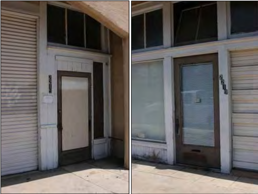
Figure 28. Contemporary view of Rose Grocery Store. Both the glass panel doors are 1920s vintage. The vertical boards above the door on the left probably sealed a transom window. The large plate glass windows probably seal original entries into the grocery. The roll up door probably would have been a barn door, such as seen on Fire Station No. 9. The larger transom window amidst the ribbon of windows above the doors is original.
