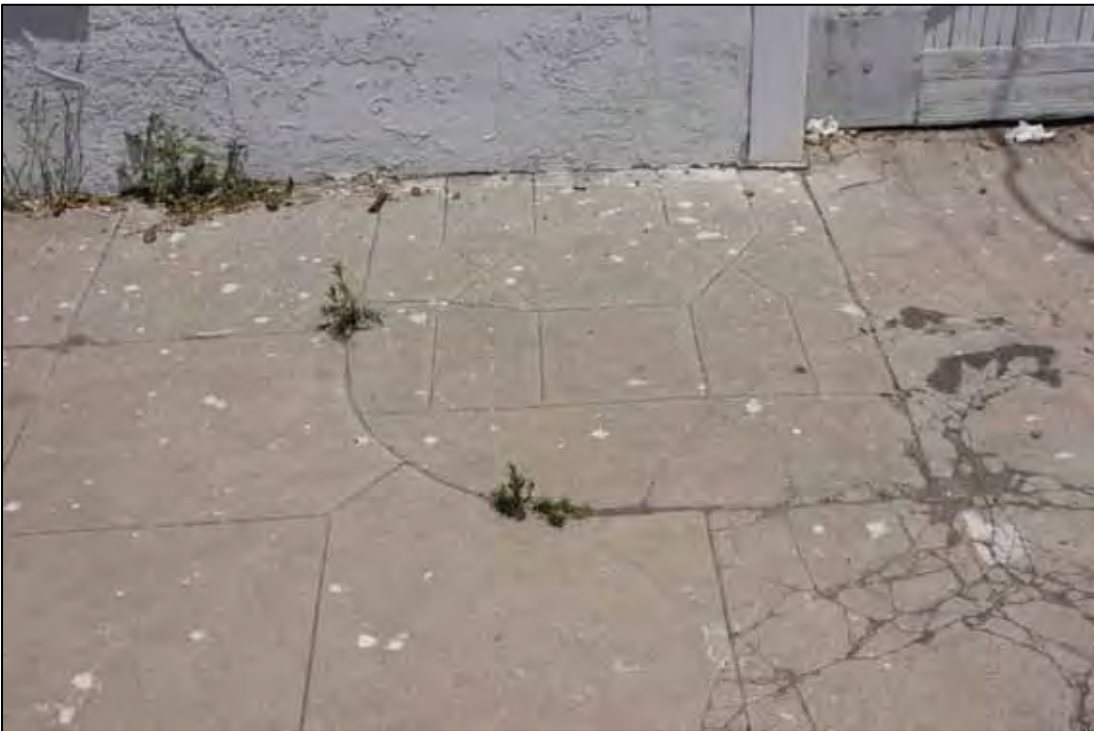
Figure 39. Contemporary photos of Burlingame Garage. By way of sidewalk archaeology, one can see the earlier walkways to the houses that preceded the Burlingame Garage on this location. The crushed concrete at the lower right was caused by a heavy truck associated with the garage history. Elsewhere on this sidewalk are marks left by the early gasoline pump and signage. These features are included in the South Park Commercial District.
