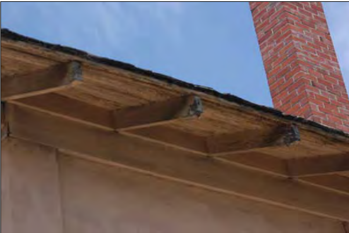
Figure 24. Contemporary views of Fire Station No 9. The modern electrical power equipment does not detract from the architectural integrity of the fire station. Note that only slight weathering of the rafter tails has occurred and this can be treated.
