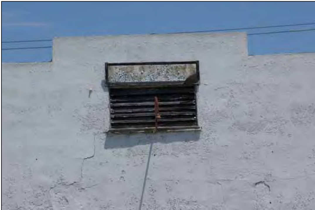
Figure 38. Contemporary photos of Burlingame Garage. The barn door and horizontal louvered attic vent are classic livery stable barn features that transitioned into early automobile garage architecture in the early 20 th century. Survival of these original architectural elements are significant examples of a scarce automotive commercial architecture that is almost extinct in San Diego. Care should be taken to repair and retain these important architectural elements.
