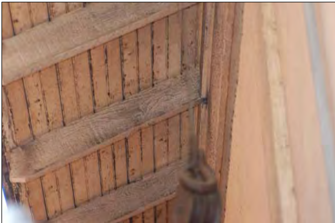
Figure 23. Contemporary views of Fire Station No 9. Details of how the 12:1 wood double hung windows relate to the exposed eaves and rafters. The pulley system in the lower photograph appears to be original too and may have enabled the firemen to move equipment down the north side of the building.
