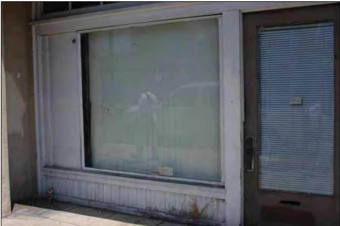
Figure 30. Contemporary view of Rose Grocery Store. The window on the left is not original, although the portal is most likely original. More careful examination would be needed to determine if the vertical boards were added after an original barn door had been removed. Conversion from the original door probably occurred during the 1940s.
