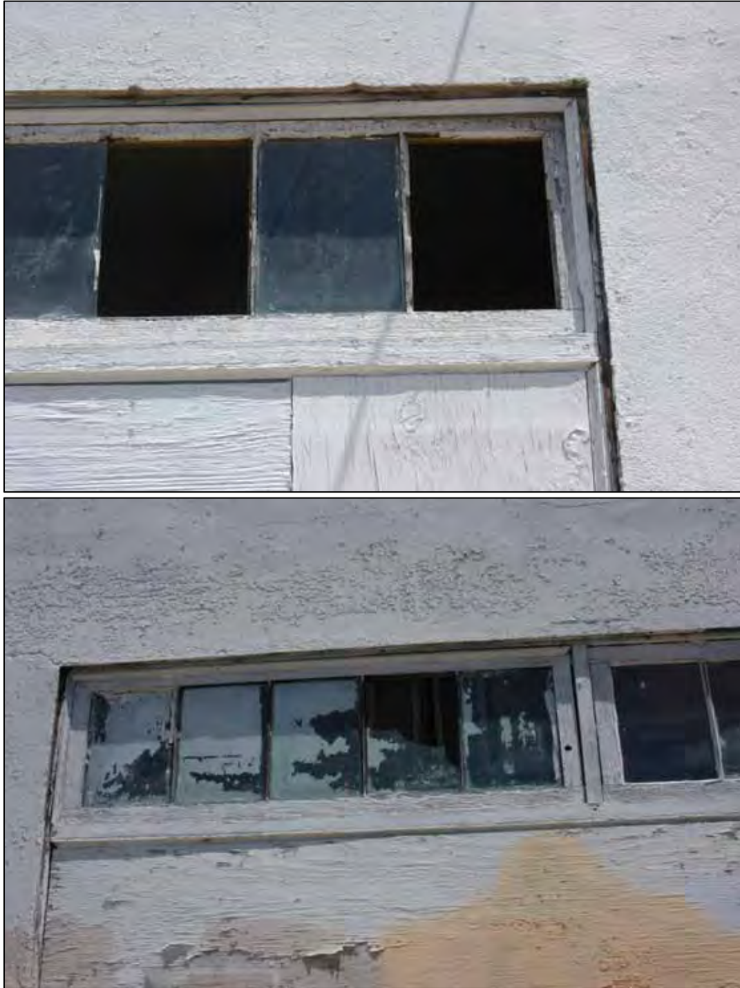
Figure 37. Contemporary photos of Burlingame Garage. Survival of the original windows and wood frames is amazing. Although the plywood board over the window is not original, it essentially mothballed the window and preserved the portal. When restoring this window system, care should be taken to retain the original frames and glass.
