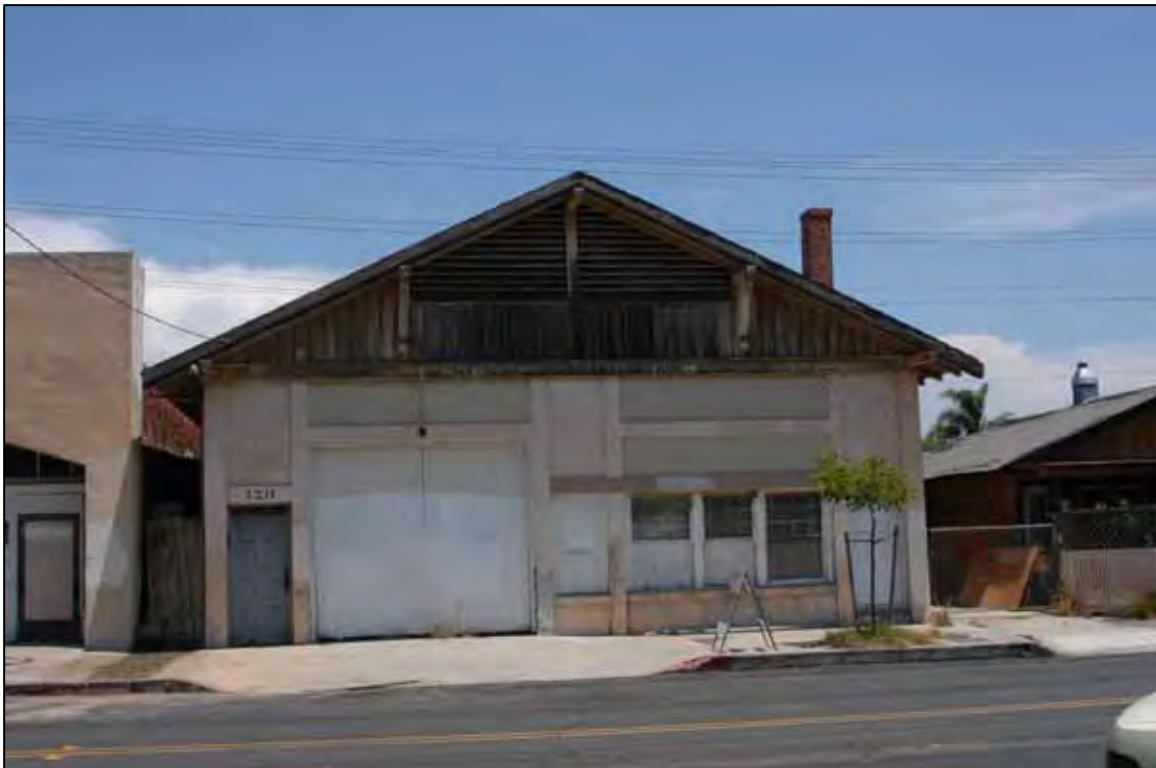
Figure 25. Contemporary views of Fire Station No 9. Note the reddish hollow clay tiles on the wall between Fire Station No. 9 and the Rose Grocery. Both buildings were built with this technology, although the fire station has a steel reinforced cast concrete frame that supported the tiles. Modern paint now obscures the brick façade over the tiles.
