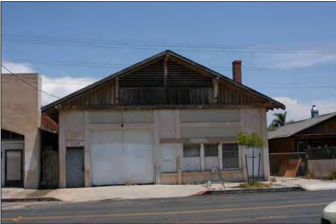
Figure 18. All the architecturally defining characteristics of this building survive. Note the barn doors are original. The door portals and windows are correct, although the doors are new. Restoration would be relatively simple.
