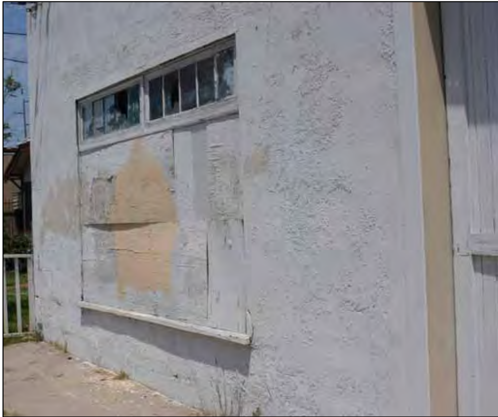
Figure 36. Contemporary photos of Burlingame Garage. Although the stucco and wood show weathering and the windows have been boarded up, the building exhibits high integrity. The original barn doors are remarkable and should be preserved. The ribbon of windows above the primary window are mostly intact and the glass could be easily repaired.
