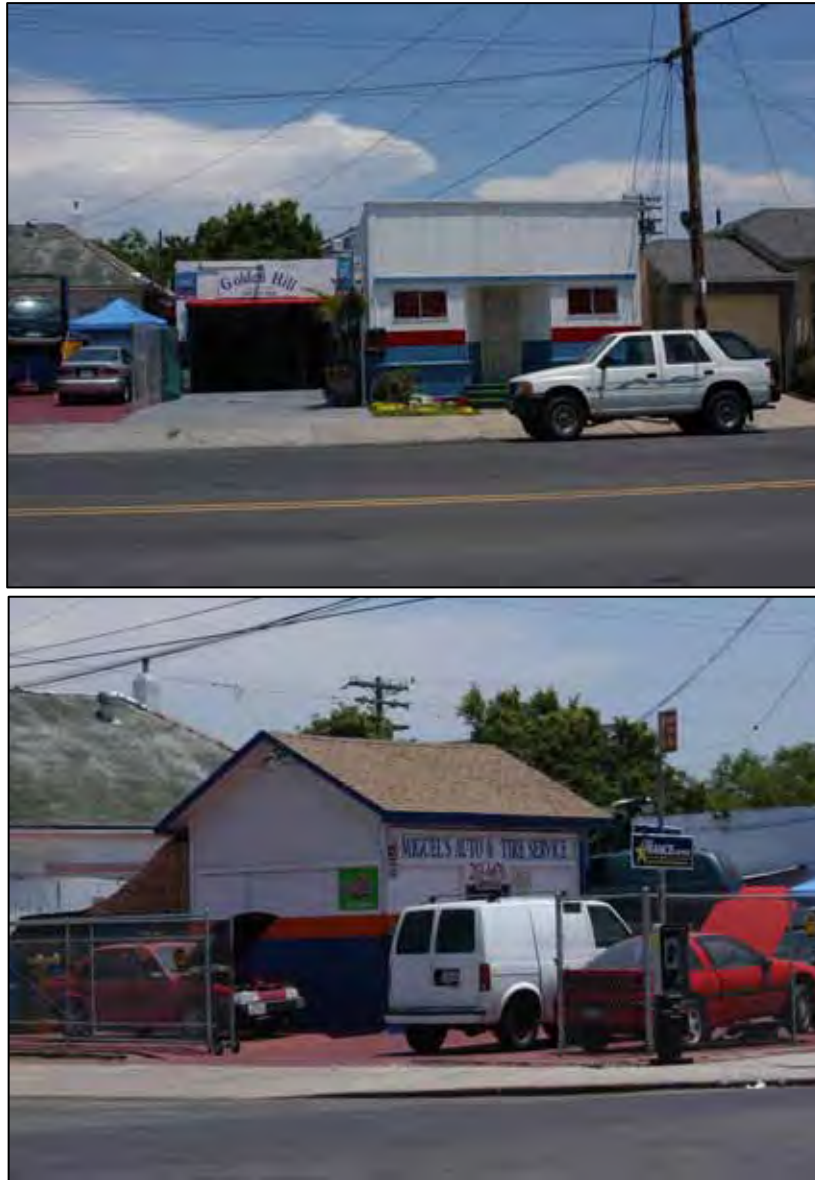
Figure 16. Contemporary views of Munter and Munter Gas Station. Note: the top photo is not part of this nomination, but is part of Miguel's Auto & Tire Service that occupies the site today. The lower photo shows the Munter and Munter office.
