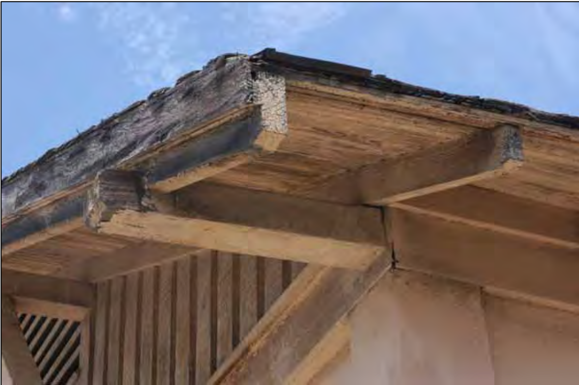
Figure 22. Contemporary views of Fire Station No 9. Note how all the original architecturally defining features have survived so well over the years.
